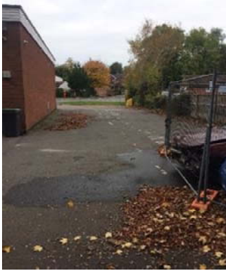
Photo 7 - Poor line marking
