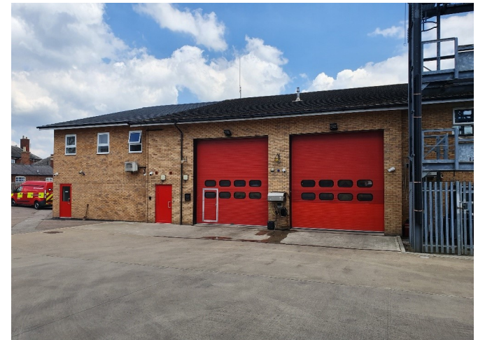
Lutterworth Station Extension
