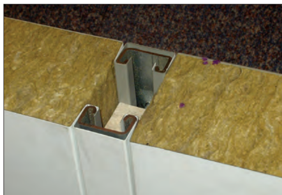
Figure 17: Insulated core panels – internal panel
